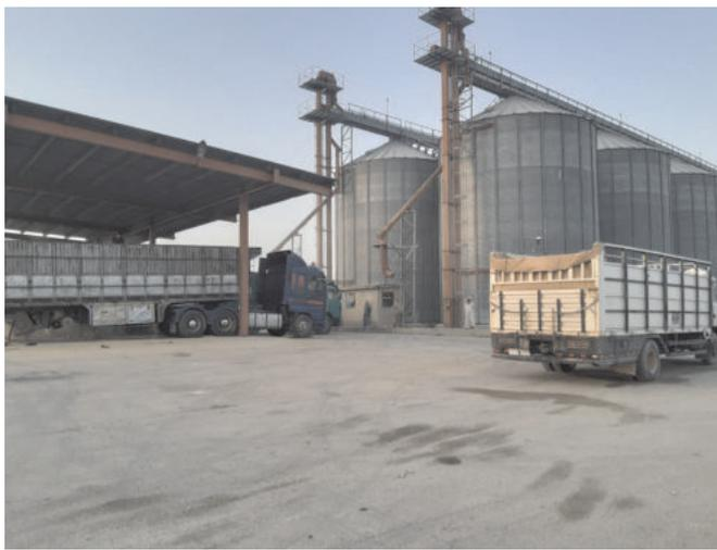
*After the quality check the harvest is dropped into a pit underneath the ground from where it is moved into the big Silos by electronic suction control.*
